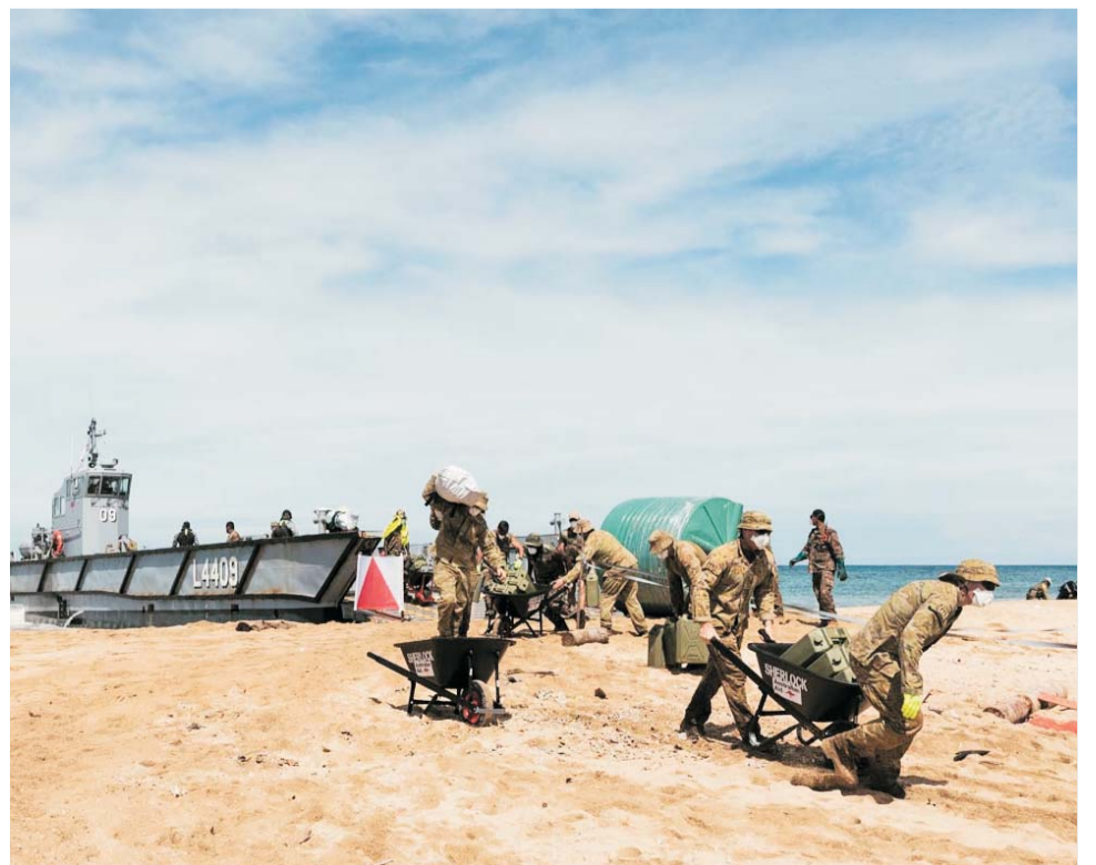
NZ Defence staff helping to rebuild Ha'apai. (Credit: Solo Savelio)
