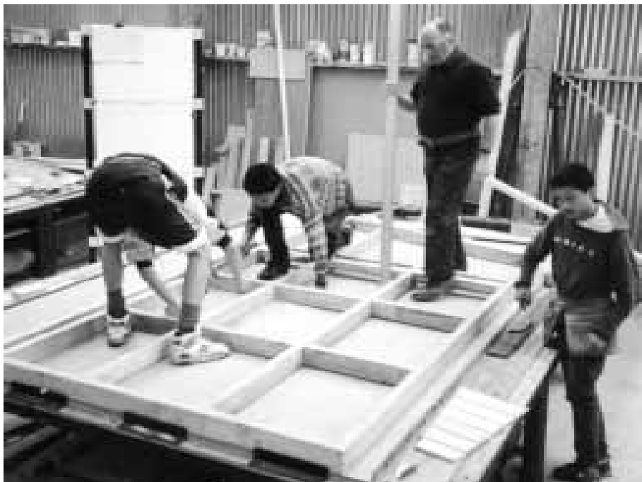
Just Housing Project: building a house panel
