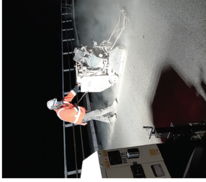
Concrete cutting an expansion joint during a night closure
