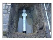
The crew will relay the wastewater lateral from the wastewater main in the road to the 'inspection point'. An 'inspection point' is where the public and private sections of the pipe meet.
